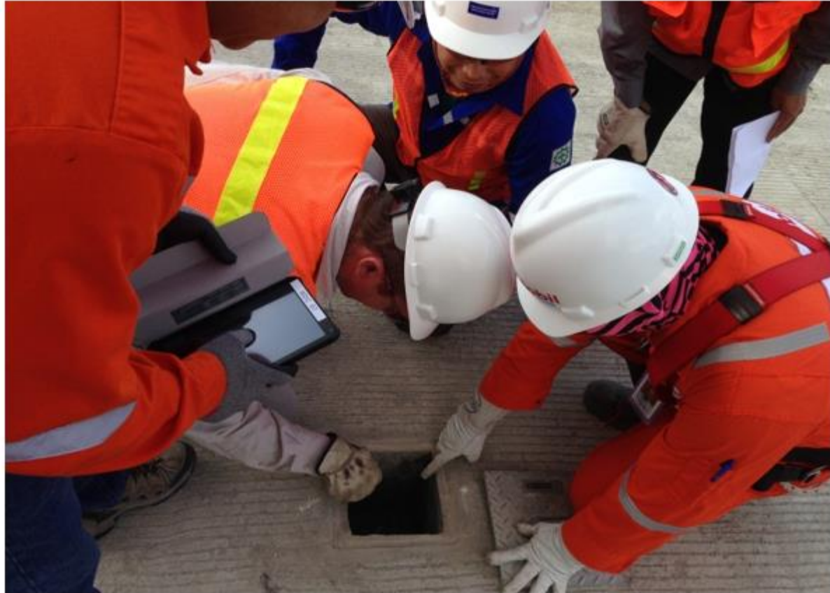
Mechanical Completion Walk Down of Earthing Subsystem
